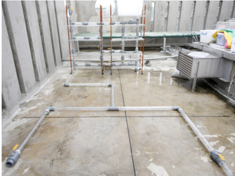
Figure 14. The experimental testbed for evaluating the PipeProbe system. 51 transparent tubes formed a 3-D non-uniform grid testbed. 21 valves with yellow handles were also installed. By opening and closing different valve combinations, different capsule flow paths and test scenarios were generated for evaluating the PipeProbe system.
