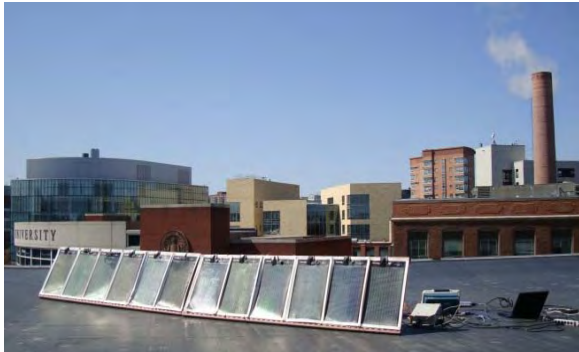
Figure 10. Picture of PV system experimental set-up at Northeastern University, Boston.
