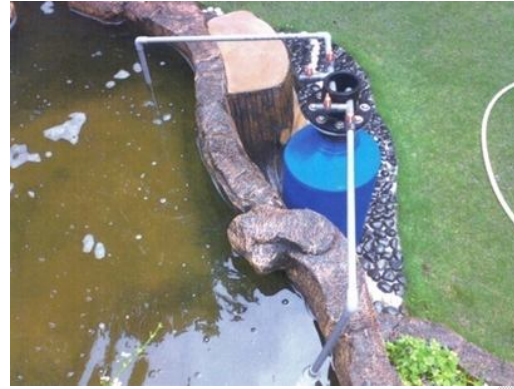
Figure 4a: Floating micro-bead bio-filter. Figure 4b: Floating micro-bead bio-filter in the koi pond.
