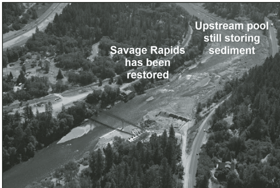
Figure 8. Sediment conditions at Savage Rapids Dam as of July 2010.
