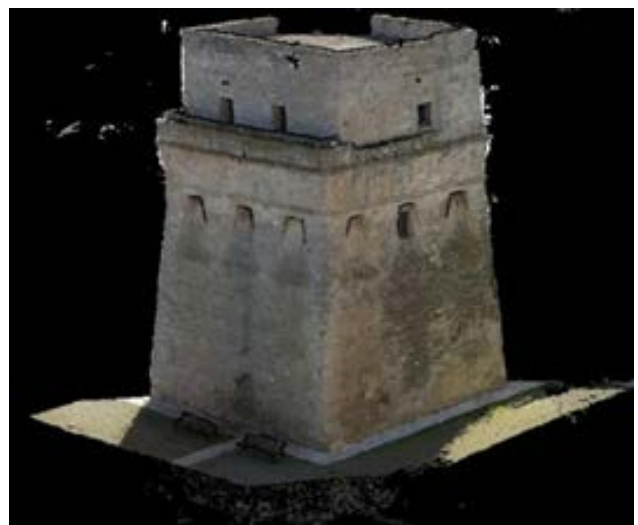
Figure 9: Point cloud model from drone shooting
