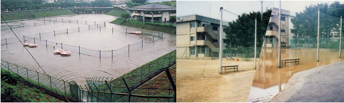
Figure 2 Tennis court and school playground equipped for water storage during excess rainfall
