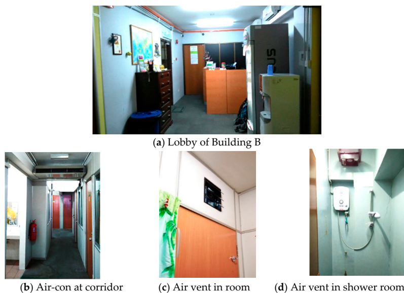
Figure 7. Building condition in Building B.
