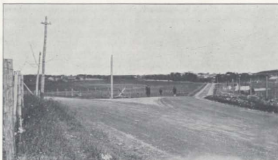
NEW ROAD TO MOUNT CASHEL FROM OLD PORTUGAL COVE ROAD.
