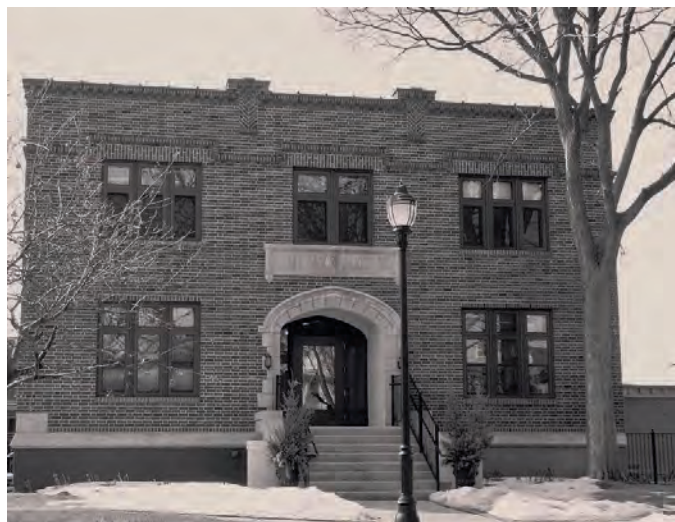
Figure 3: Maternity Hospital located at 301 Penn Avenue North in Minneapolis, MN.
