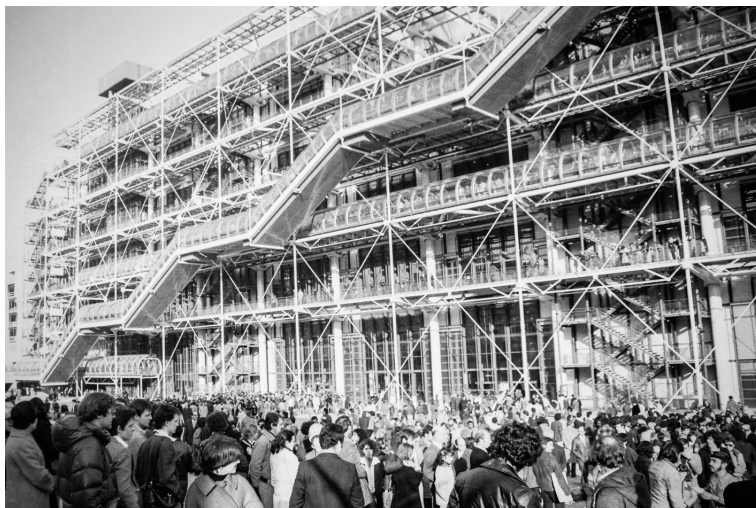
Figure 2.11: The Centre Pompidou in paris from 1978. The casted steel gerberettes Can be seen connecting the trusses and the facade structure. Photo by Upic/Tonyjoe.Gardener.
