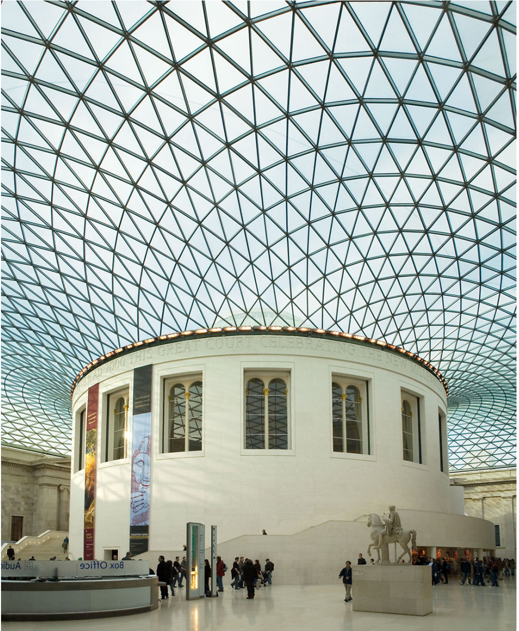
Figure 2.33: Roof structure defined by Chris Williams, where the shape is defined such that the horizontal thrust is concentrated to the corners. Photo by Andrew Dunn, http://www.andrewdunnphoto.com/ . Licensed under CC-BY-SA 2.0.
