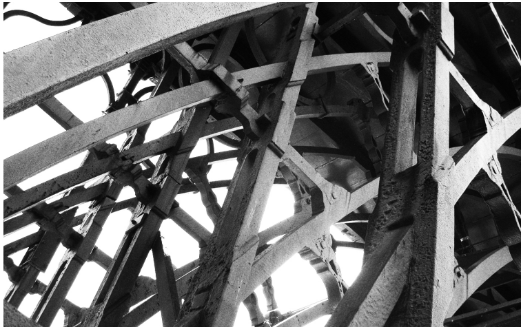
Figure 2.8: The first bridge build with iron is located in Shropshire in England and is called the Iron Bridge. The bridge is built using joining techniques from traditional wooden crafts. ©Photo by Uncle Silver.
