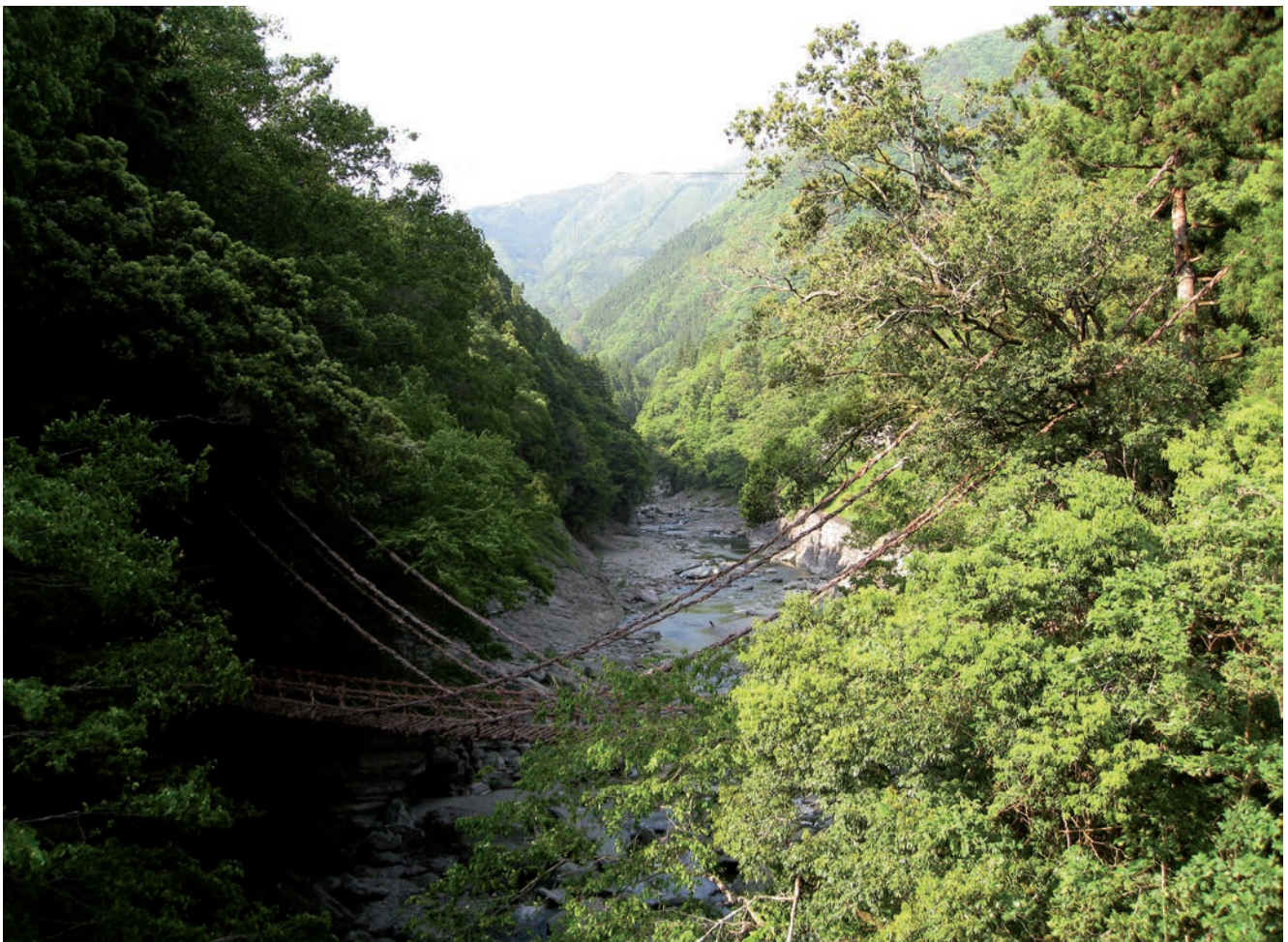
Fig. 17. Kazura Bashi bridge. Famous suspension bridge over the canyon Iya stream. In the west from Tsuguri mountain – prefecture Tokushima, Sikoku). This bridge is made of Actinidia auguta (kind of kiwi vine) and is 45 long, 2 meter wide, and is suspended 15 meters above streams. It was only access over the deep canyon into the mountainous area in those days. The bridge is changed every three years. Designated as a national and prefectural significant folk cultural assets), phot. U. Myga-Piątek • Most Kazura Bashi – słynny wiszący most nad kanionem rzeki Iya, na zachodzie gór Tsuguri, wykonany z pnącza kiwi Actinidia auguta . Most jest odnawiany co trzy lata i jest wliczany do narodowych dóbr kultury, fot. U. Myga-Piątek
