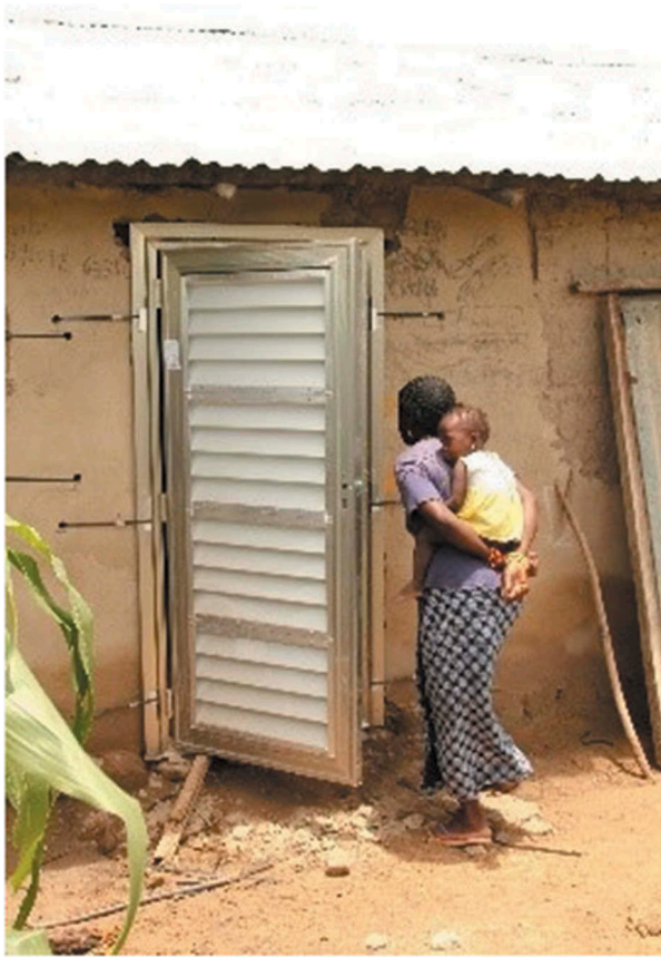
Figure 4. Prototype mosquito-proof door which allows ventilation.
