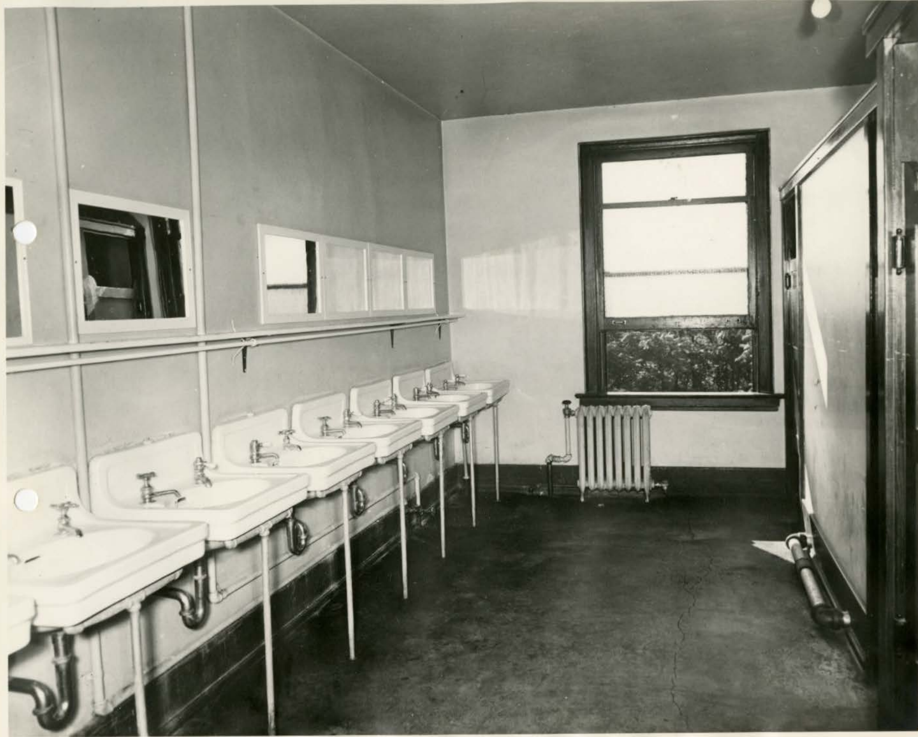
LAVATORY AND SHOWER ROOM, POTTER HALL DORMITORY.
