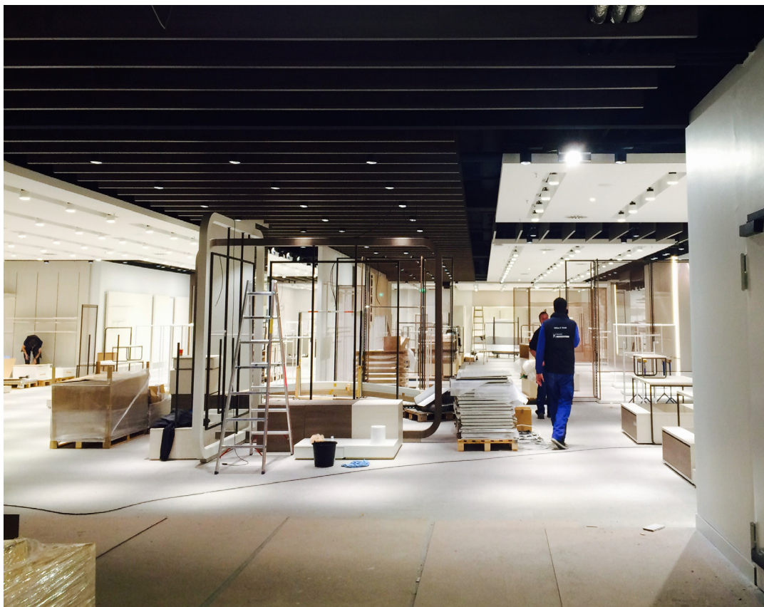
Mock-up under construction
