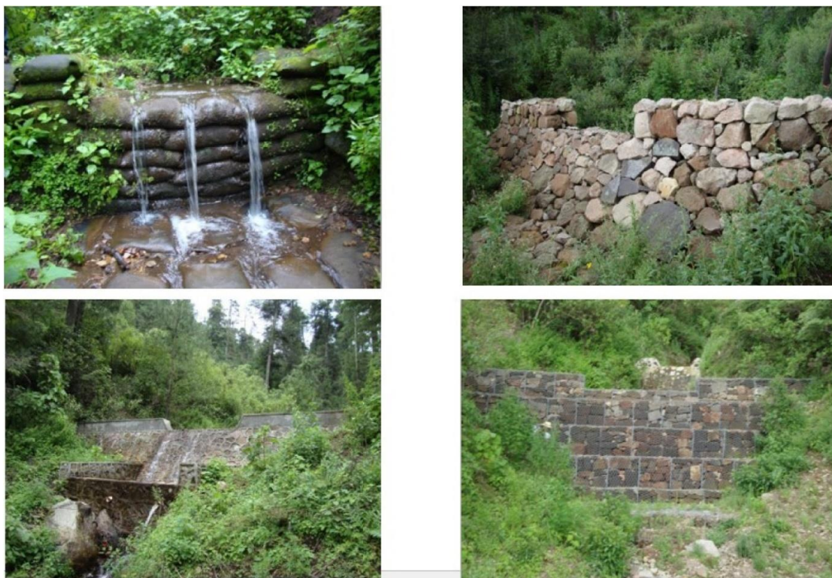
Figure 4.13: Examples of four different check dams (from Abbasi et al., 2019 [pp. 689]).
