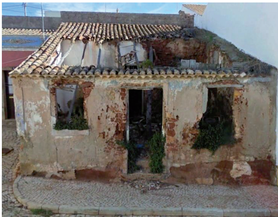
Figure 7. Vila do Bispo, typical house of vulnerability class A built with raw materials: load-bearing walls made with adobe bricks, doors and windows with lintels, and wooden logs supporting a tiled roof over a bed of reeds. Source: Google Earth.
