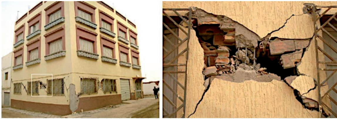
Figure 18. Imzourem, short column effect in a three-story residential block of vulnerability class C (grade 4). On the right, a detail of the damage is shown. Source: P Murphy.
