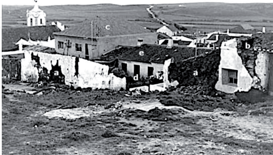
Figure 3. Vila do Bispo, general overview: (a) loss of the outer leaf of load-bearing walls and detachment of plaster; (b) partial toppling of façade wall, pulling down part of the roof; (c) good behavior of a recent construction (class B); (d) simple overturning of a freestanding masonry wall; (e) adobe house without apparent damage. Source: IPMA.
