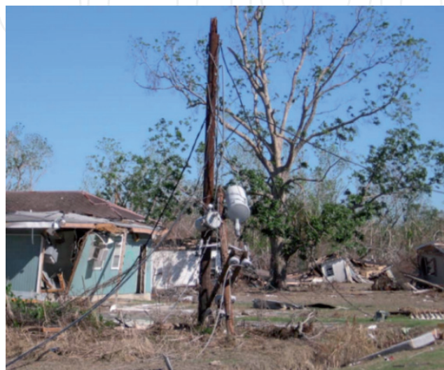
Figure 2. Damage to the electric distribution grid near Pt. A La Hache, LA.
