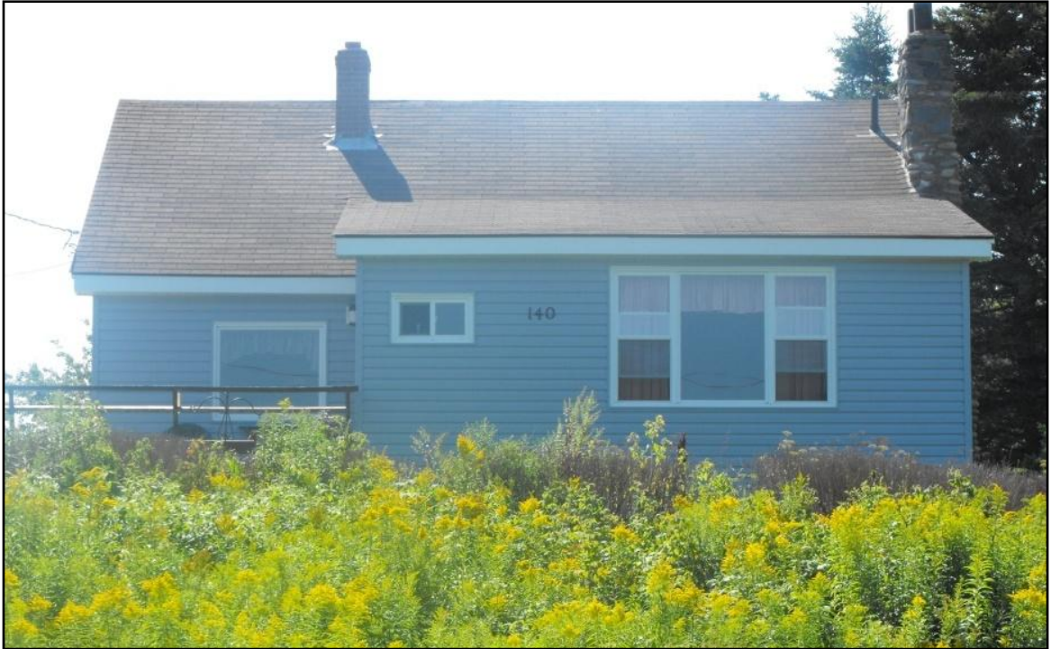
Figure 3-15: The front of the house at 140 Dyke Road, facing west.
