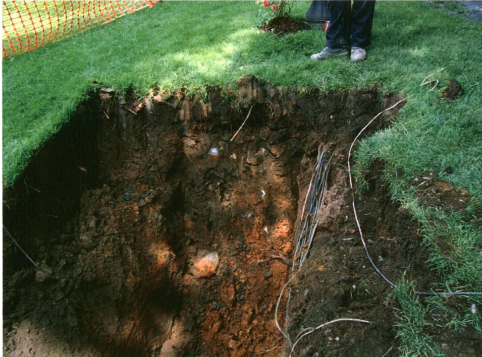
Plate 3: North edge of catch basin trench showing ironstone 0.35 metres below surface, looking north.
