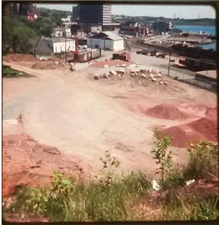
Figure 4.4. “Burial” mound under construction, June 1977. (NIP-1976, 101 80C 7-1 Harbourview. Halifax Municipal Archives)
