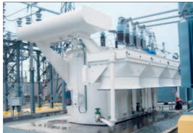
2 The transformer in (1) has been remanufactured to a fully functional state
