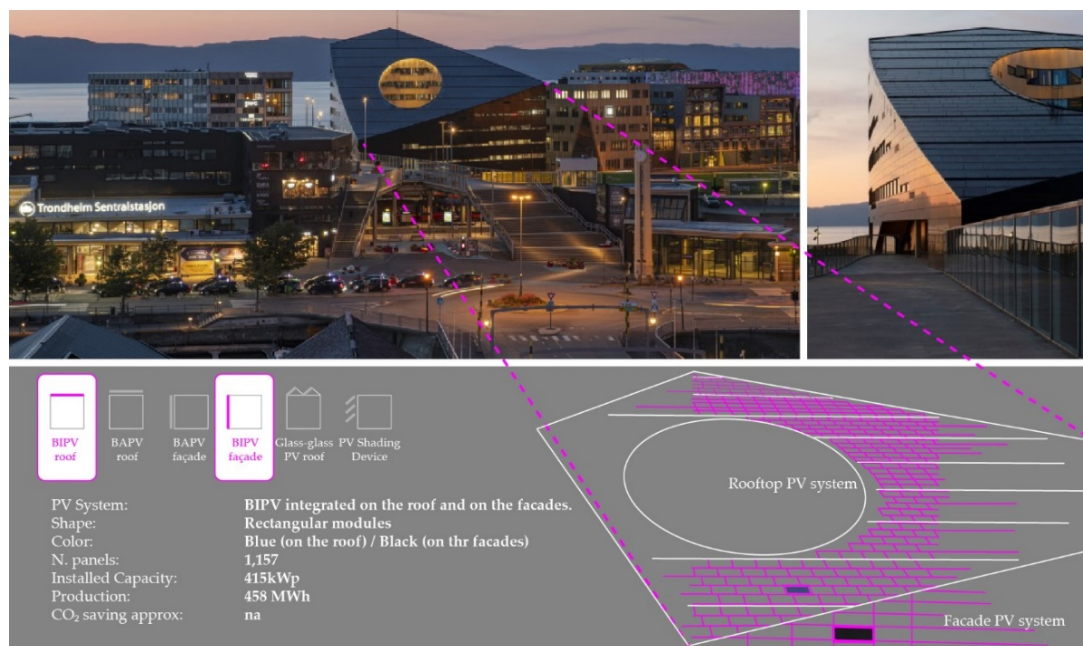
Figure 8. Powerhouse Brattørkaia (photo on top by Ivar Kvaal, with permission from Powerhouse http://powerhouse.no ) (on the top); Integration and characteristics of PV systems (on the bottom).
