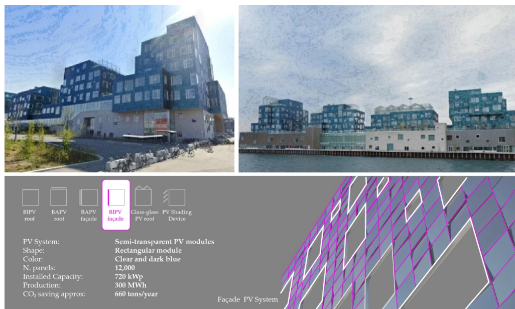
Figure 14. Copenhagen International School (a top view and elevation: Source of illustration Google Earth, Google 2020) (on top). Integration and characteristic of PV systems (on the bottom).
