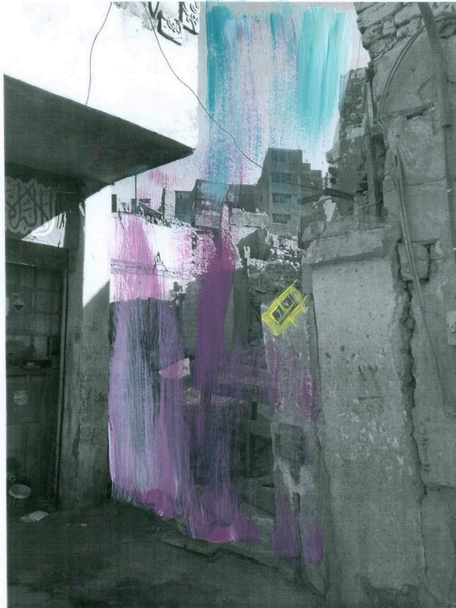
Picture of House number 1 8 : While in al-Hattaba with two of my Megawra BEC coworkers in April 2019, we discovered that this house that was demolished by its owners. The demolition took place around February 2019.
