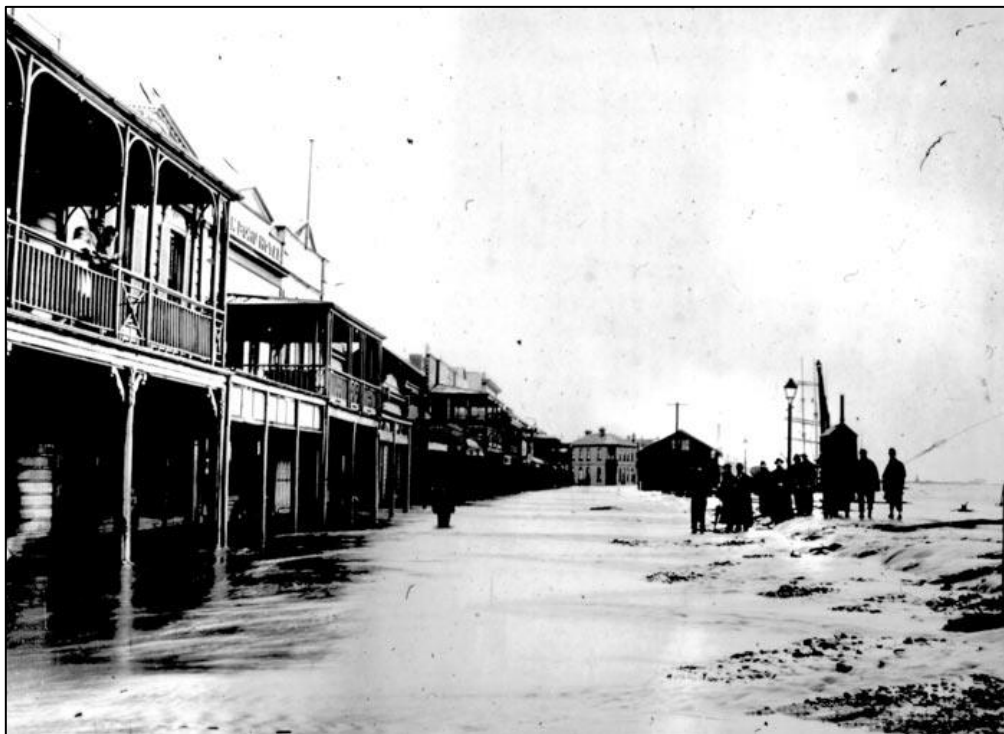
Figure 3.3 - Flooding on Mawhera Quay following the 1887 flood (McMillan Brown Library, UC)
