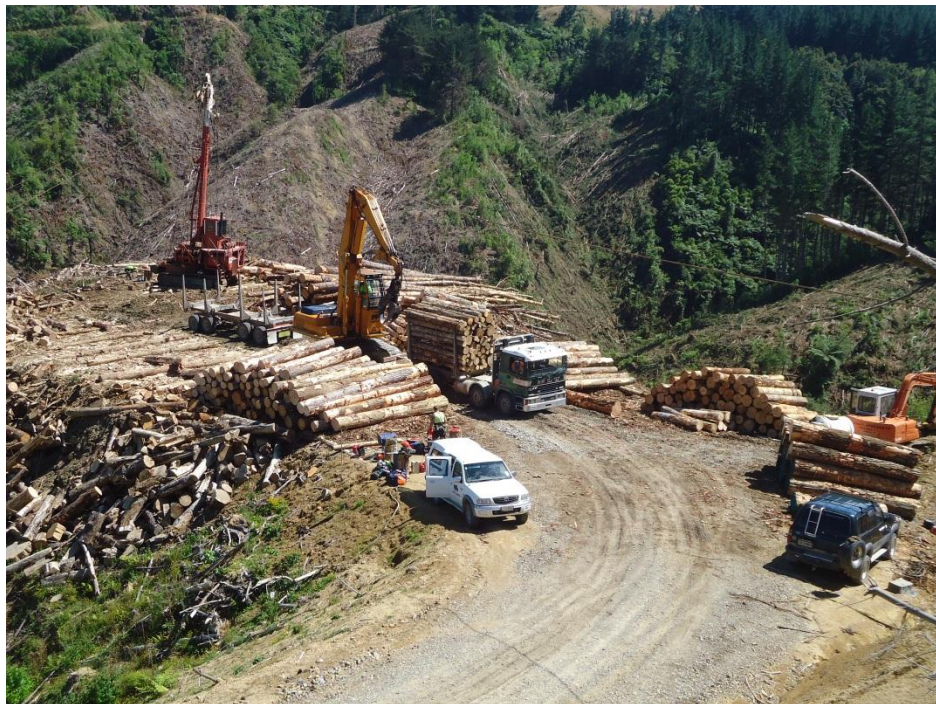
Figure 1 - A typical New Zealand woodlot cable logging landing.
