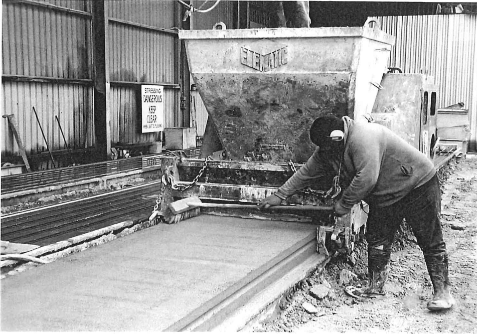
Fig. 1.14 Brooming of an extruded hollow core surface
