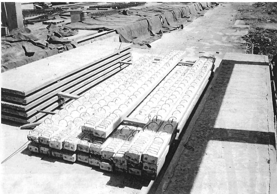
Fig. 1.5 Manufacture of pretensioned joist units (Interspan)
