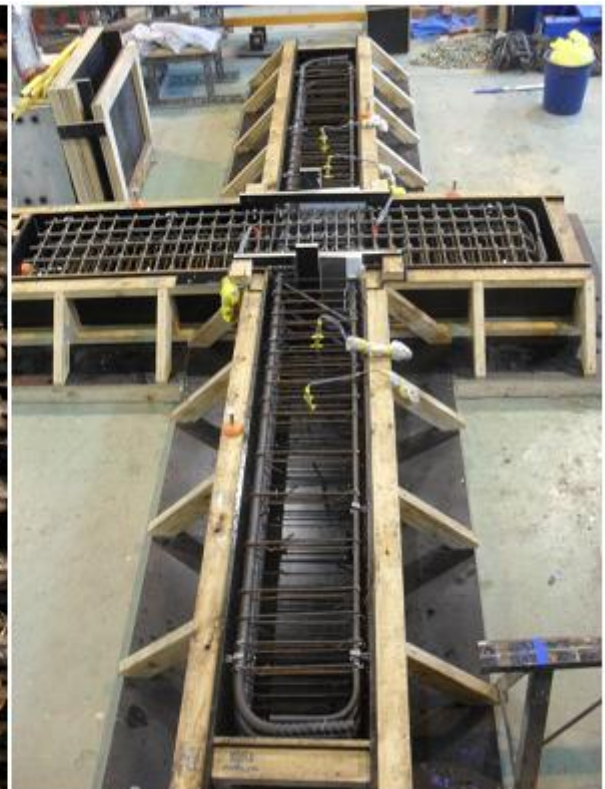
(f) Finished cage in formwork
