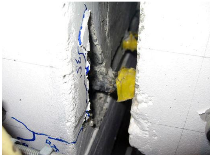
Figure 2-17: Reduced concrete cone pullout damage in specimen SB3 (Au, 2010)
