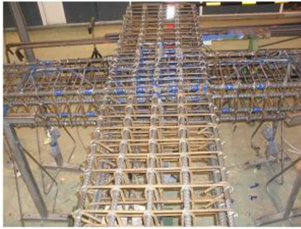
(c) Caged beam-column joint
