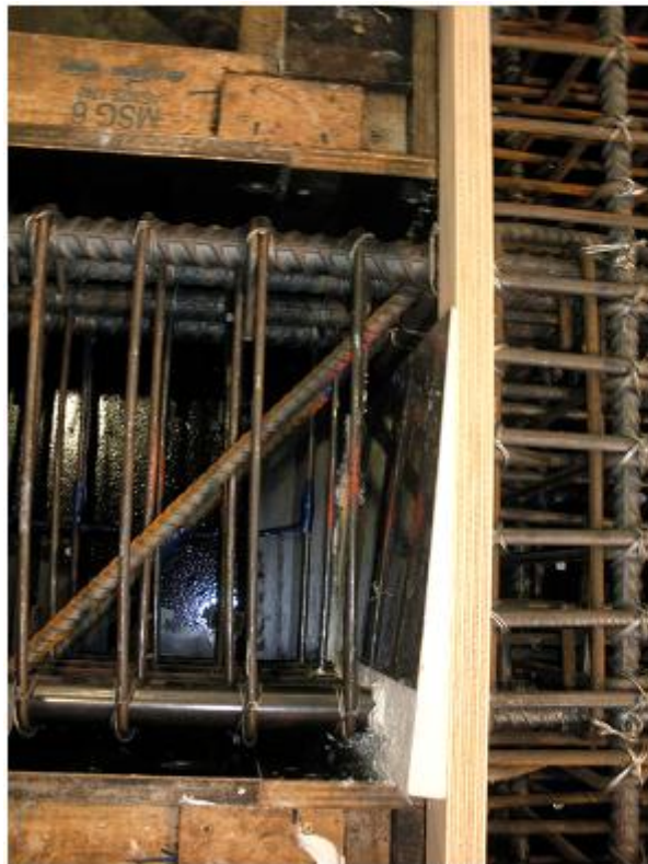
(e) Slot form and shear hangers
