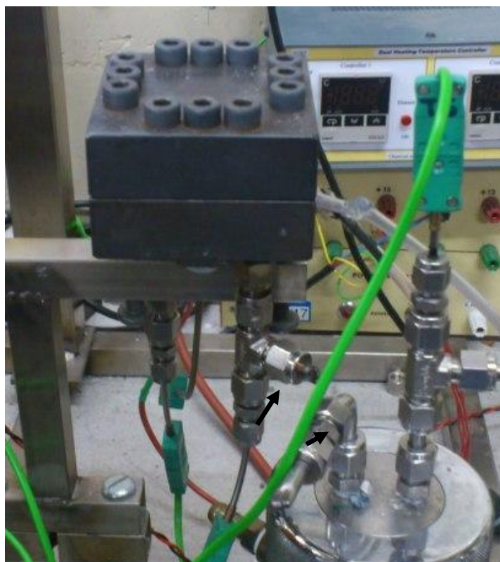
Figure 41: Arrangement of reactor showing outlet to collection pot. Note the line is separated and capped between runs to eliminate air oxidising the catalyst
