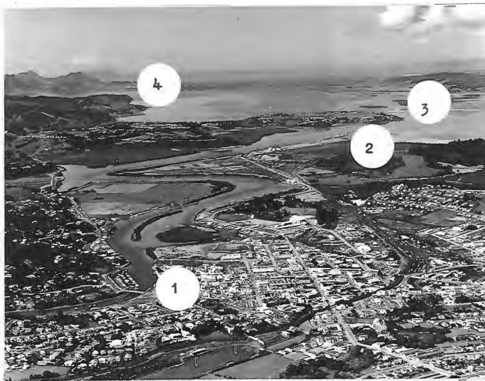
Plate XVII. Whangarei Harbour. The four separate wharf areas are widely scattered. (1) The Town Wharf used for coastal vessels. (2) Kioreroa Wharf used by overseas shipping for discharging oil, fertiliser and general cargo. (3) Portland Wharf used for shipping cement coastwise and receiving coal from West Coast (S.I.). (4) The site of the oil wharf which now serves the new refinery. Photo: Whites Aviation.
