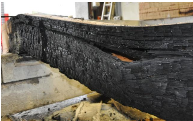
Figure 23: Test 3 beam after the test.
