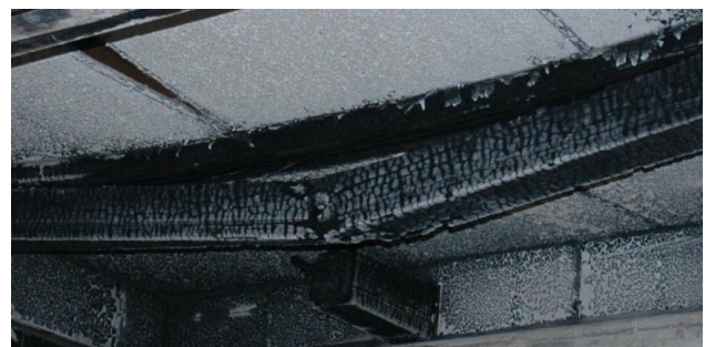
Figure 21: Test 2 beam after the test.
