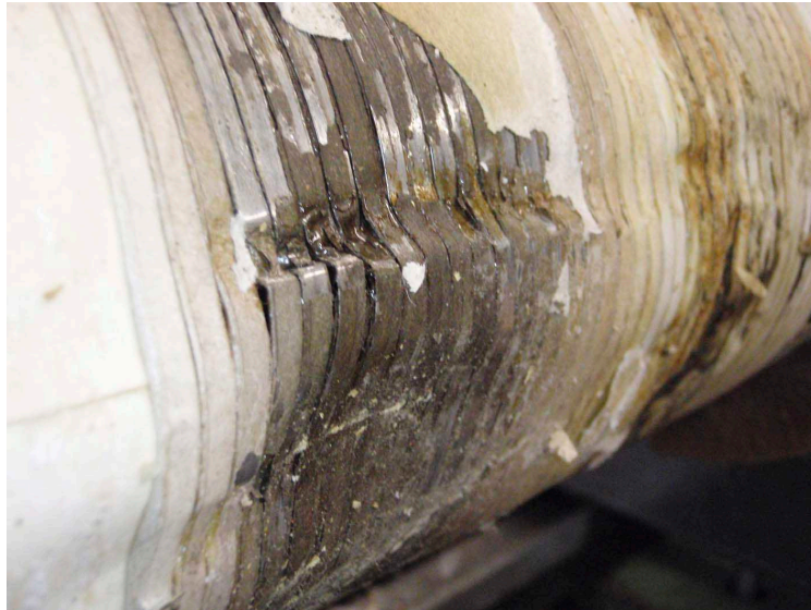
Figure 3.10 A photograph of the radial buckling that occurred on the inside windings.
