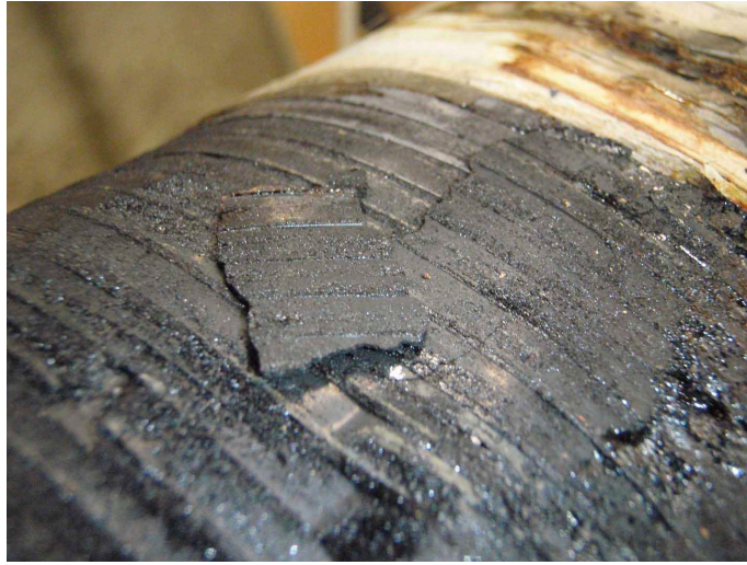
Figure 3.9 A closeup photograph of the burnt Nomex ® insulation.
