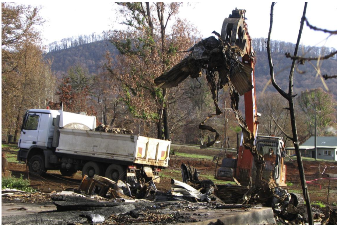
Figure 9-2 Contractors remove metal separated from bushfire waste following the 2009 Victorian Bushfires. (Photo date: March 2010.)
