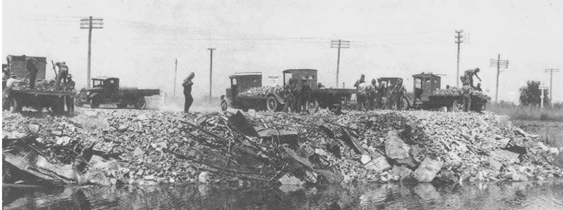
Figure 1-2 Following the 1931 Napier earthquake, rubble from collapsed buildings was first dumped into a lagoon just west of the Napier CBD (pictured) and later along the Napier waterfront (photo source Alexander Turnbull Library)
