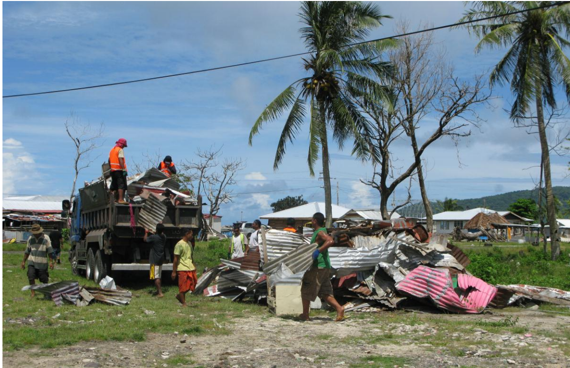
Figure 8-1 Contractors collecting bulky metal for recycling
