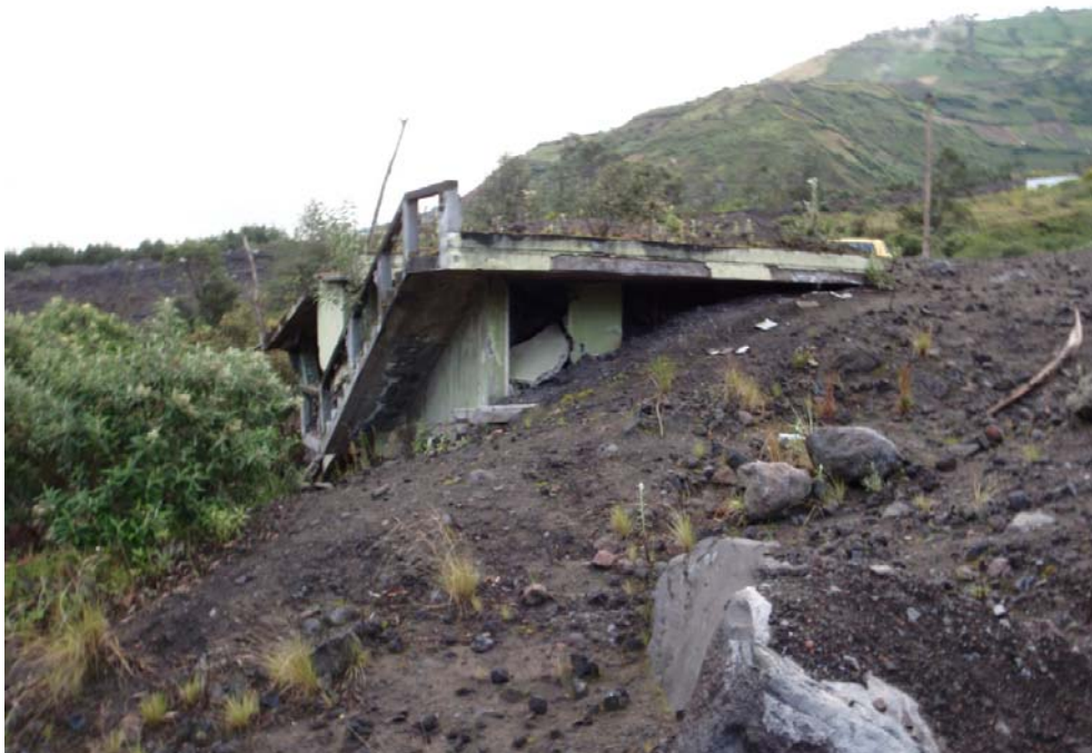
Figure 15 Area of lahar damage in Juive Chico, west of Baños (GPS 16). Upper photo: new section of road replacing lahar-damaged section. Lower photo: in same area, house buried by lahar deposits.
