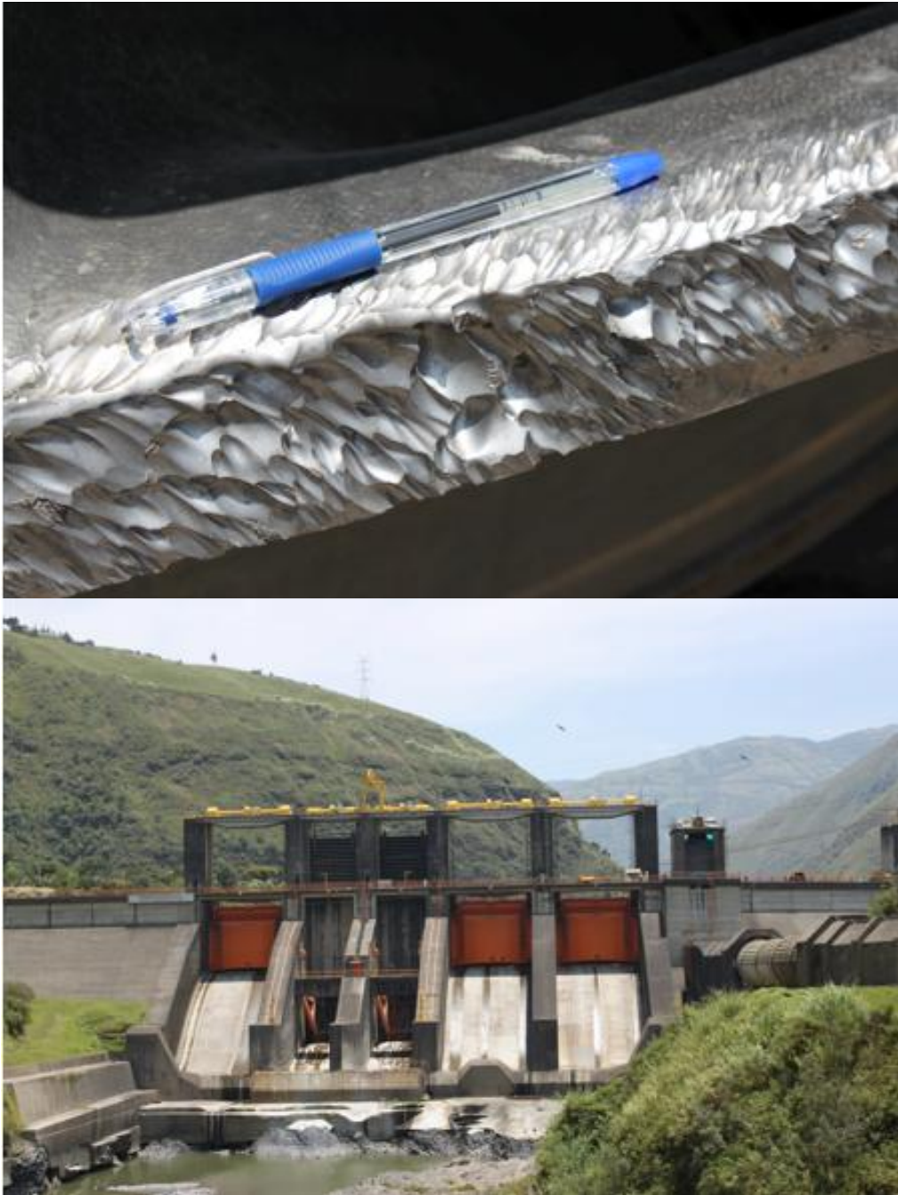
Figure 12 Above: a severely pitted turbine that has been removed from service. Below: the Agoyan Dam and its orange floodgates.
