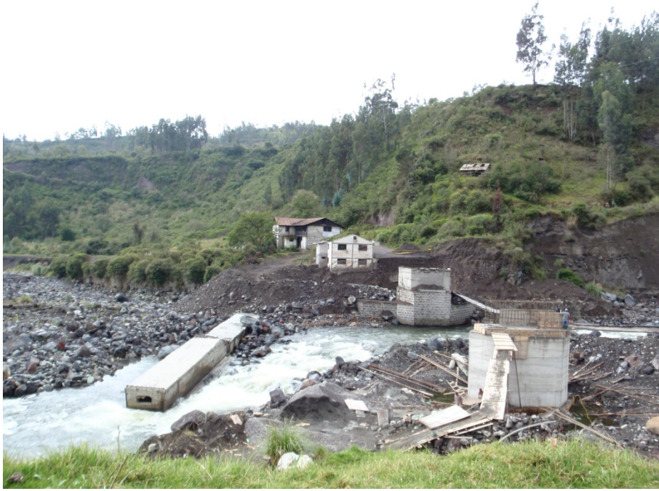
Figure 1 Bridge on Rio Palitahua washed out by lahar from Volcán Tungurahua, near settlement of Penipe, on direct route between Riobamba and Baños.
