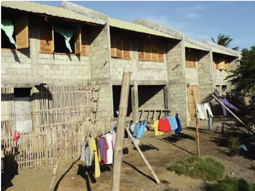
Figure 5.2 Row houses at the KABALAKA resettlement area (Photo: HPFP, 2009; Text: author).
