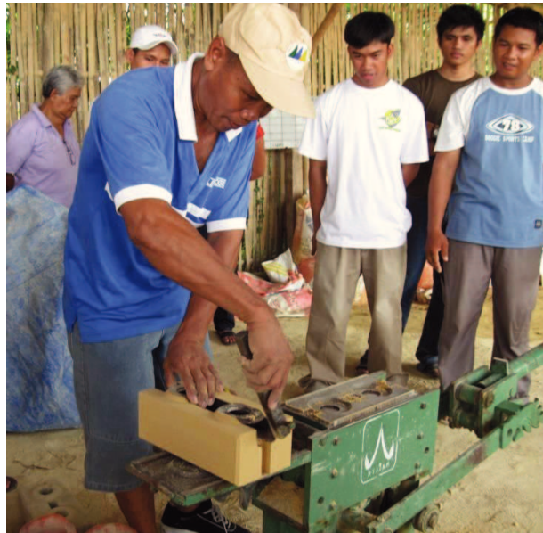
Figure 5.4 Hands-on training of CLIFF beneficiaries on Interlocking Compressed Earth Block Production (Text and photo: HPFP, 2009).
