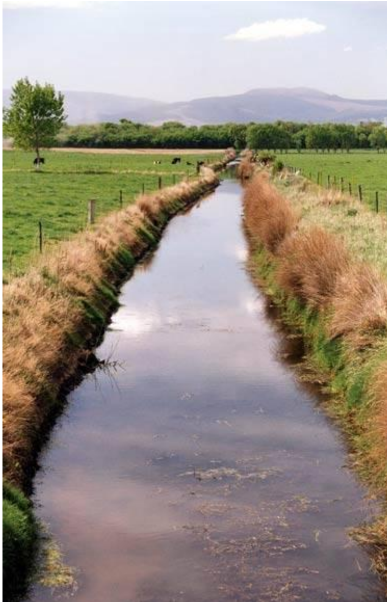
Plate 3.3 Drainage canals on the Rangitaiki are managed in conjunction with the regional district and a farmer run co-operative. Adequate fall is increasingly problematic, owing to subsidence and tectonic movement (Rangitaiki Plains, eastern Bay of Plenty, New Zealand)
