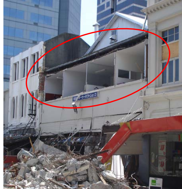
Figure 4: Facade loss attributed to building crushing
