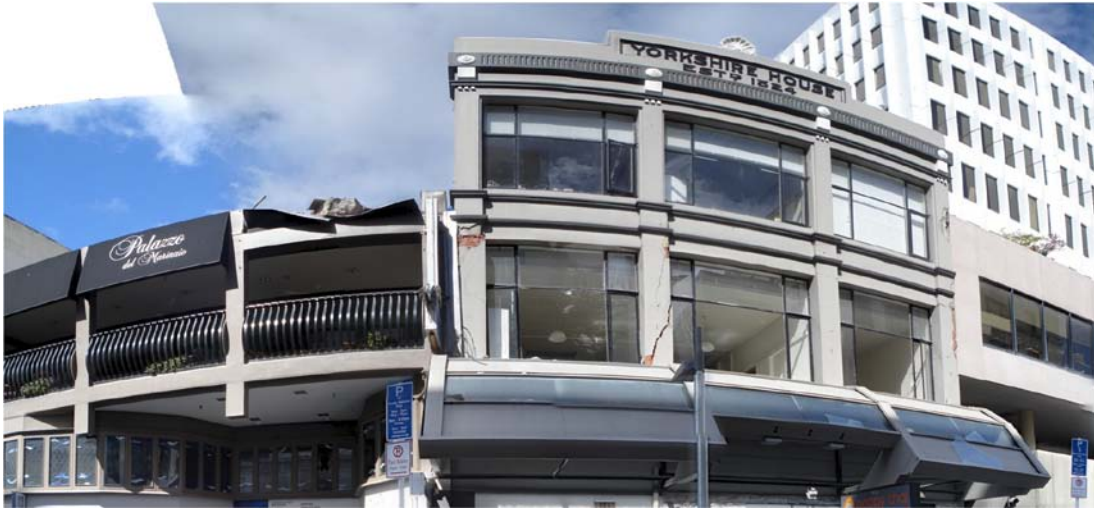
Figure 5: Pounding damage caused by buildings with greatly differing heights. Note image is distorted due to panoramic photography
