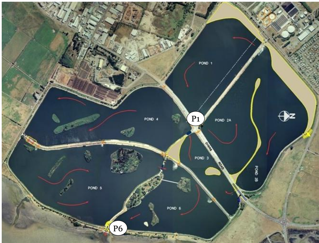
Figure 2-2. Aerial Photograph of Oxidation Ponds at CWTP, NZ.
