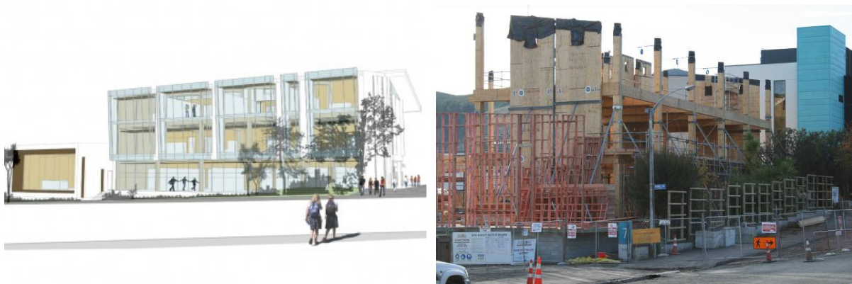
Figure 2.23 NMIT Building, Nelson (Photo courtesy Aurocon and M. Newcombe)
