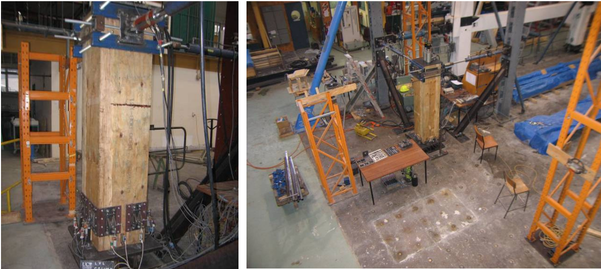
Figure 5.6 Details of loading jacks and view of test setup
