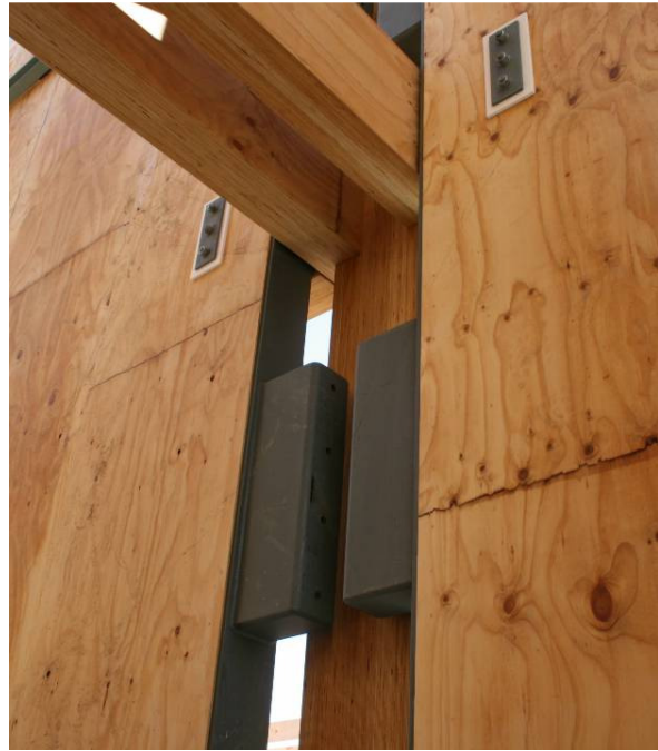
Figure 4.14 UFP connections in practical building application (NMIT Building, Nelson; photo courtesy M. Newcombe)
