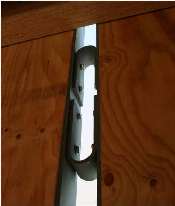
Figure 4.14 UFP connections in practical building application (NMIT Building, Nelson; photo courtesy M. Newcombe)
