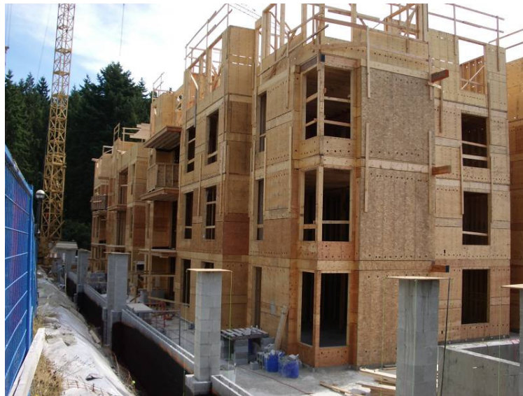
Figure 1.2 Multi-storey timber building in Canada with plywood shear walls (Courtesy: A. H. Buchanan)
