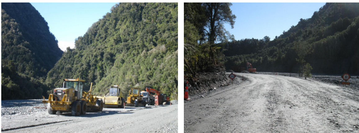
Photo 14 and Photo 15 Road works on Franz Josef Glacier access road
