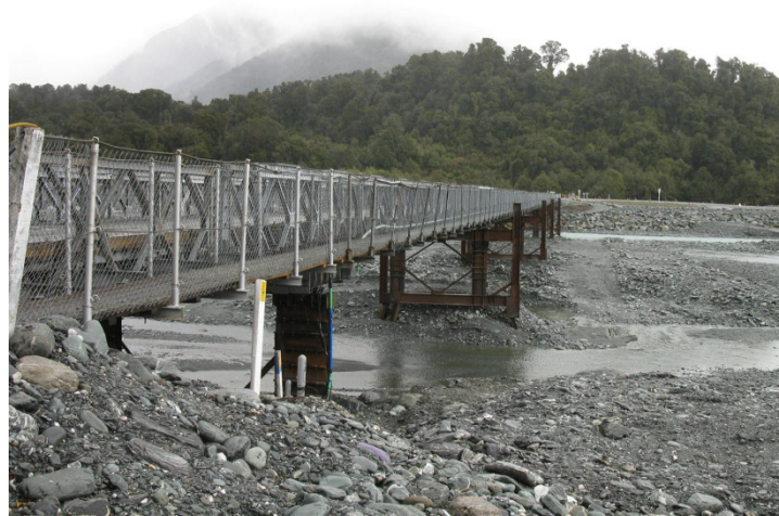
Photo 9 The Waiho River Bridge & aggrading river bed
