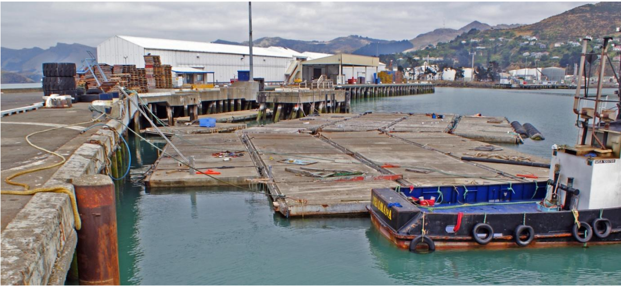
Figure 1.8: View of Z wharf pontoons site, Lyttelton Port, facing west.
