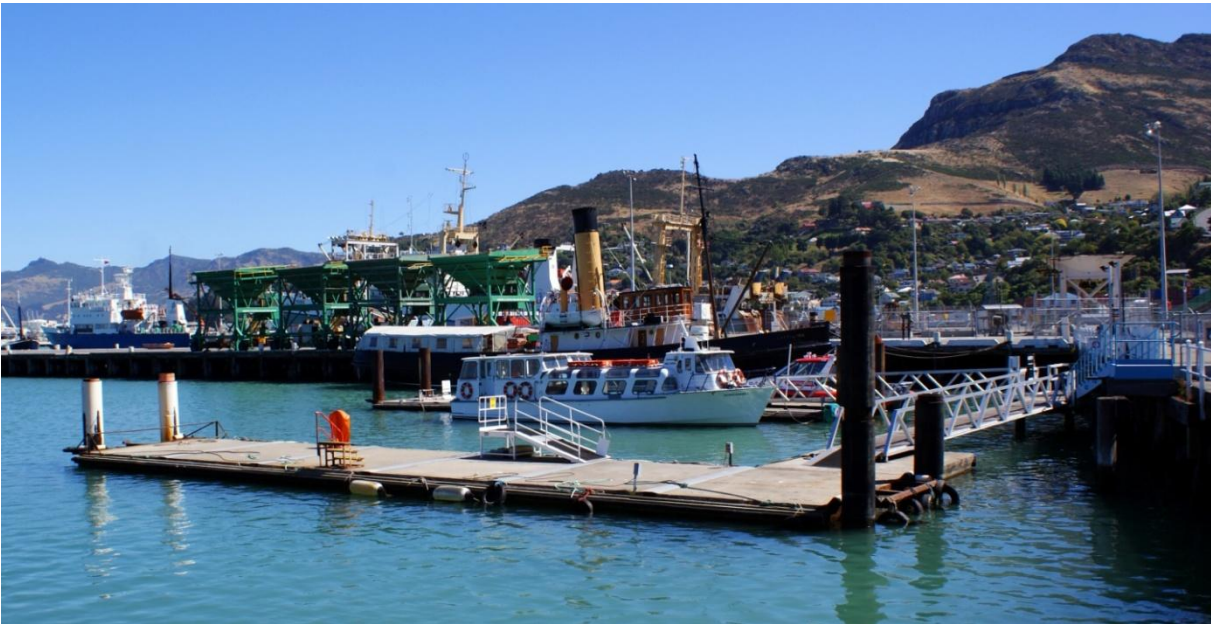
Figure 1.7: View of A&B pontoons site, Lyttelton Port, facing west.
