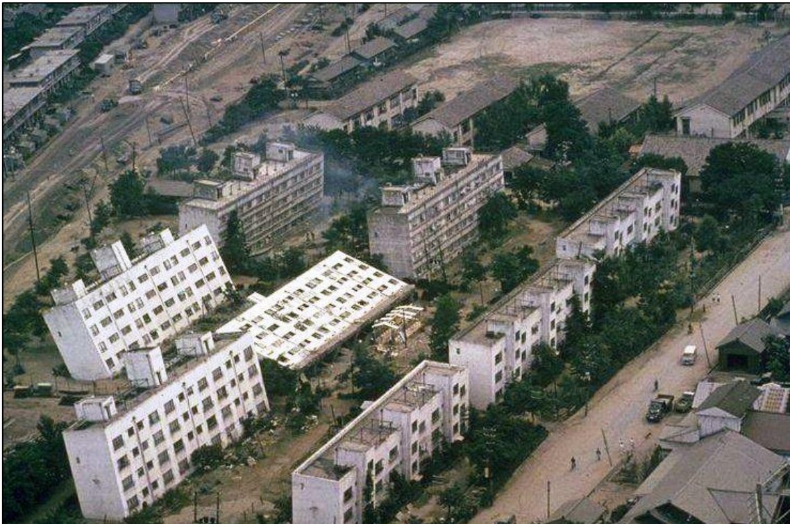
Figure 3.1: Toppled apartments, Niigata 1964 (US National Geophysical Data Center (NGDC) 1964).
