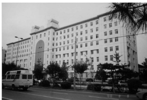
Fig. 2. Story-increased structure after construction in China [12]
