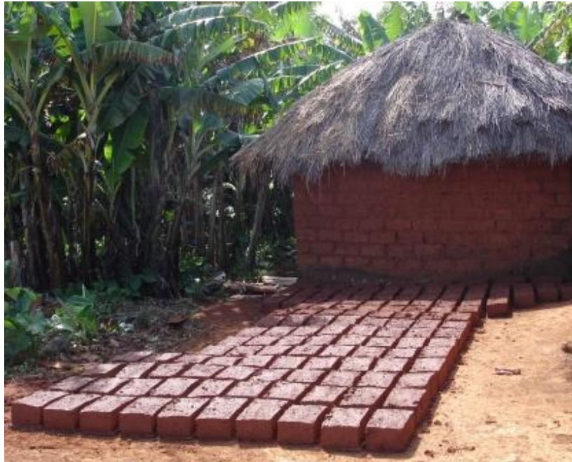
Figure 6 Mud bricks drying in the sun
