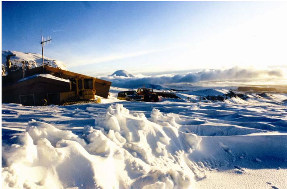
Figure 10 Tukino Lodge, extreme winter conditions
