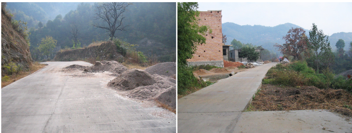
Left: Sand piled on the road by local people to block tour buses. Right: Unfinished road construction owing to the villager's interference.
