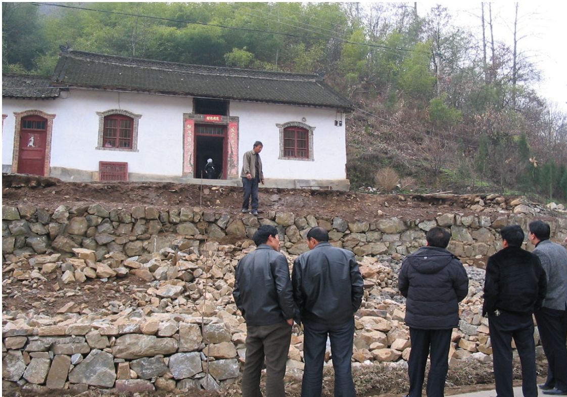
Plate 19: Quarrel at site of family hotel construction
