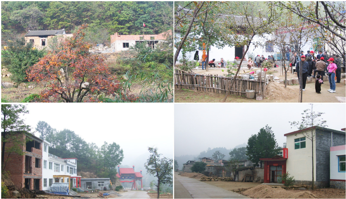
Top: A new house being built as a family hotel (left). Family Hotel 2 was hosting a group of tourists (right). Bottom: The nearly completed construction of a new family hotel (left) and Family Hotel 5 (right).
