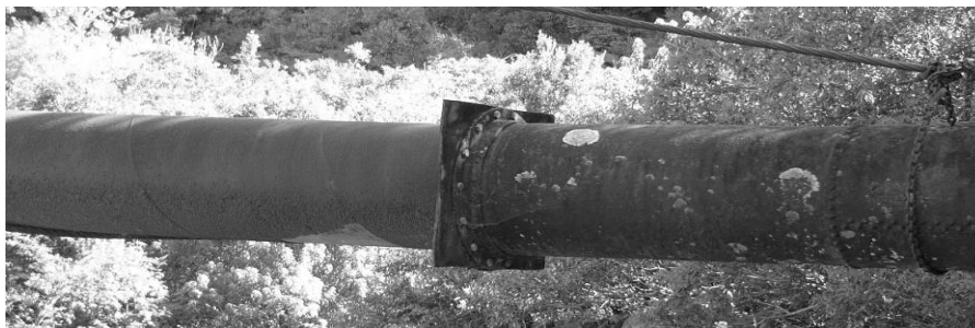
Figure 4: Spiral welded pipe abutting original riveted cast iron pipe
