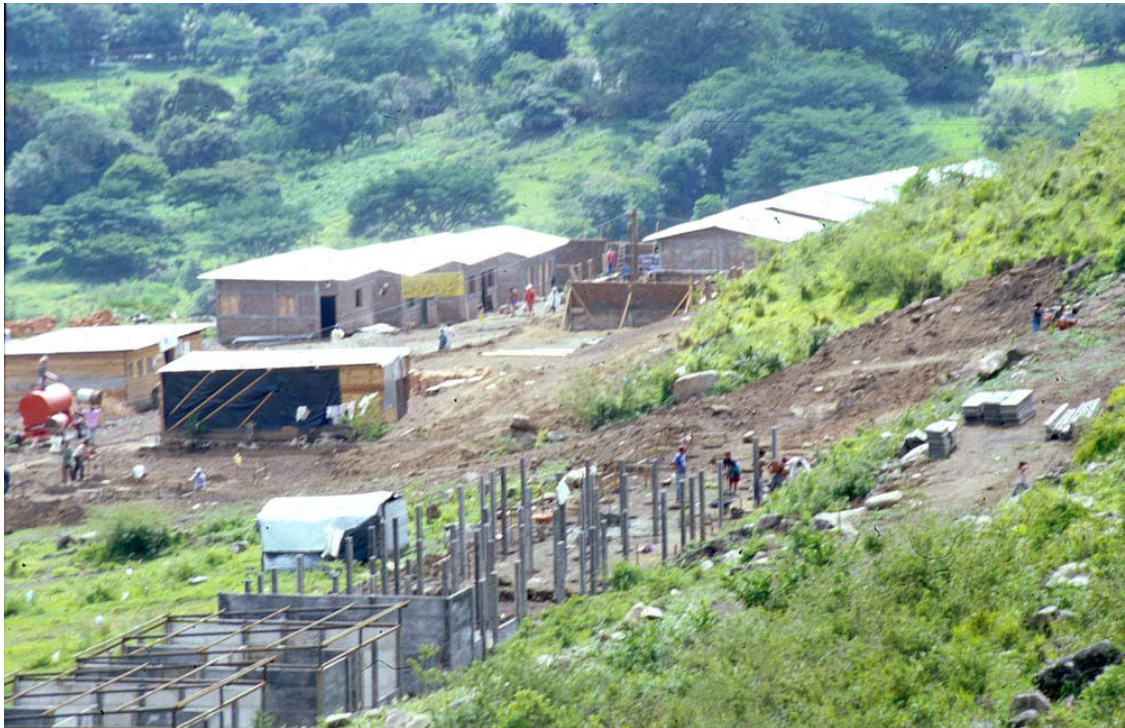
Figure 7.6 Construction at El Mirador Source: Julie Cupples
