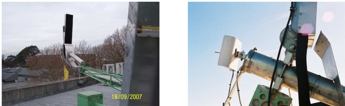
Figure 3.7. The boom extension and target with plumbing and auto-tracking head.
