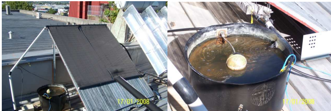
Figure 10.20 a & b. Pool mat solar thermal system, radiator and storage tank, January 2008.
