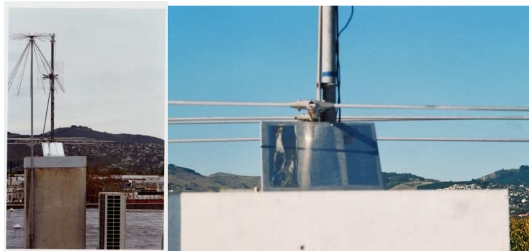
Figure 8.2 a & b. The first test panel (TP#1) on top of the old boiler chimney C block roof CPIT September 2003.
