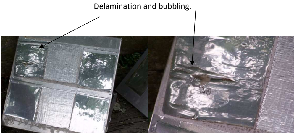
Figure 8.52 a & b. AP#2 25 th January 2006, progressive failure of the 3M substrate.
