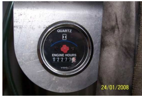
Figure 5.20. The CP engine runtime indicator.
