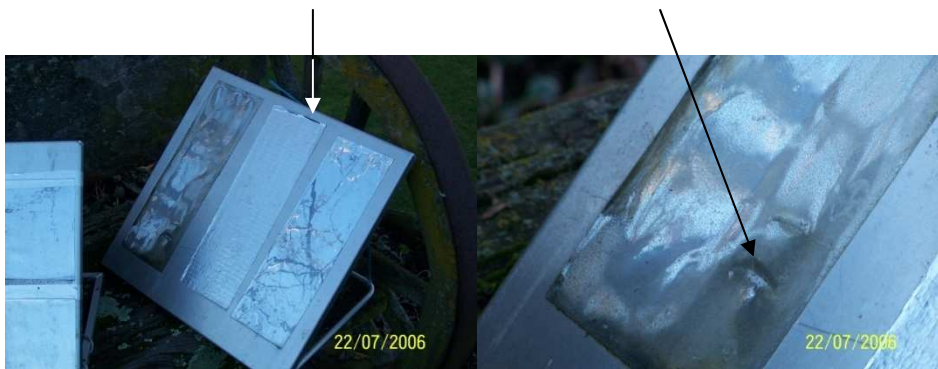
Figure 8.24 a & b. TP#2 taken 22 nd July 2006, showing the 3M substrate Mylar cracking failure and some lifting of the Clear Dome substrate top edge.
