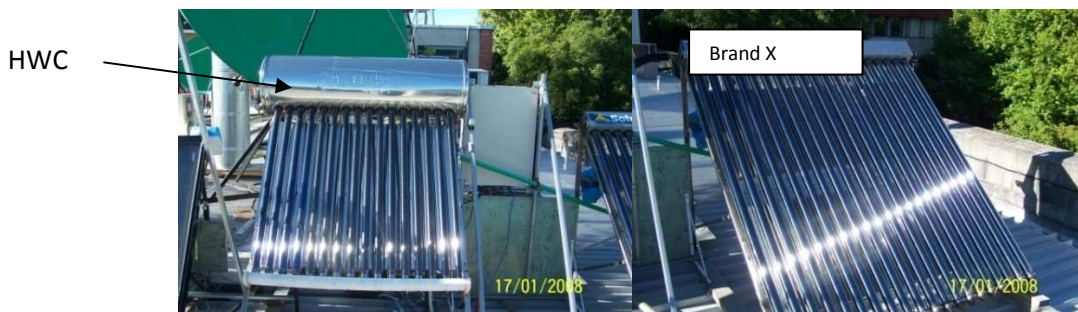
Figure 10.6 a & b. Showing 38 mm diameter evacuated tubes and 55 mm diameter evacuated tube heat pipes.
