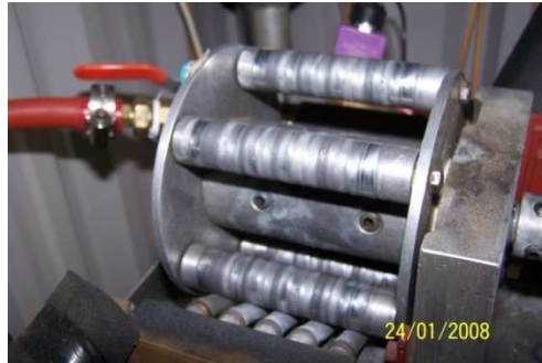
Figure 5.13. Peristaltic pump roller assembly and bypass pipework in background.
