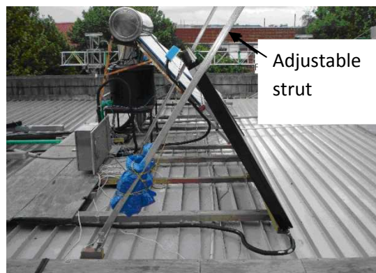
Figure 10.9. Showing sliding mounting brackets for flat plate collector.
