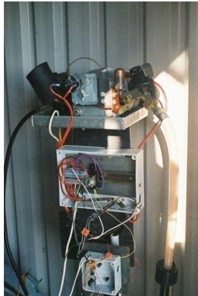
Figure 5.11. The CP controller upgrade in progress.
