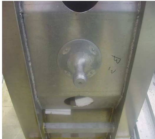
Figure 3.19. A mirror's rear mounting detail.
