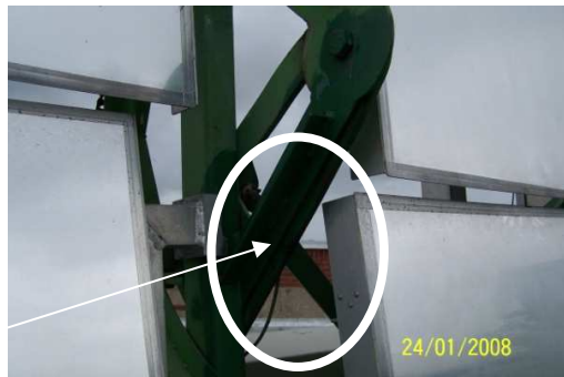
Figure 3.22. Y axis frame pivot without bottom strengthening gusset.
