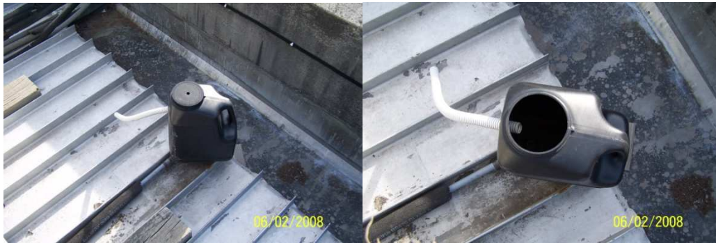
Figure 4.3 a & b. Hot water exhaust dumping container.
