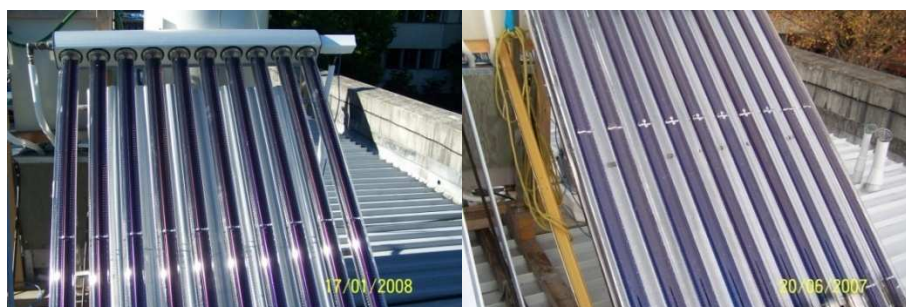
Figure 10.8 a & b. Evacuated tube finned heat pipe technology.
