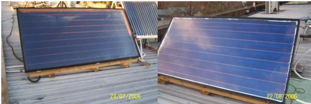
Figure 10.4 a & b. Urethane and Rockwool insulated flat plate collectors.
