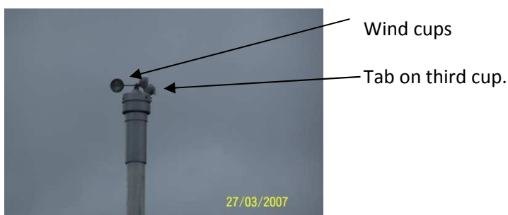
Figure 9.7. Wind anemometer in normal operation, March 2007.
