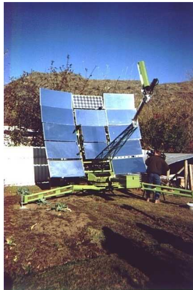
Figure 1.1. The SET in its original installation in Queenstown, 1997.
