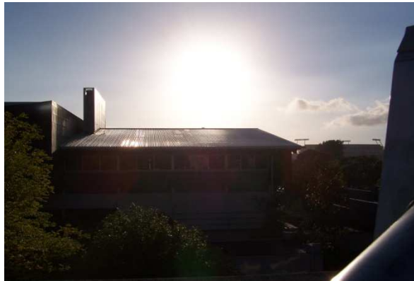
Figure 1.4. The third floor extension to E block, to the east side of the SET, sunrise (0752) on 17 th February 2006, with the SET boom to the lower right of picture.
