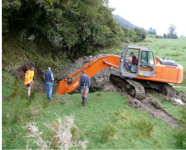
Figure 25: Digging of the trench in progress.
