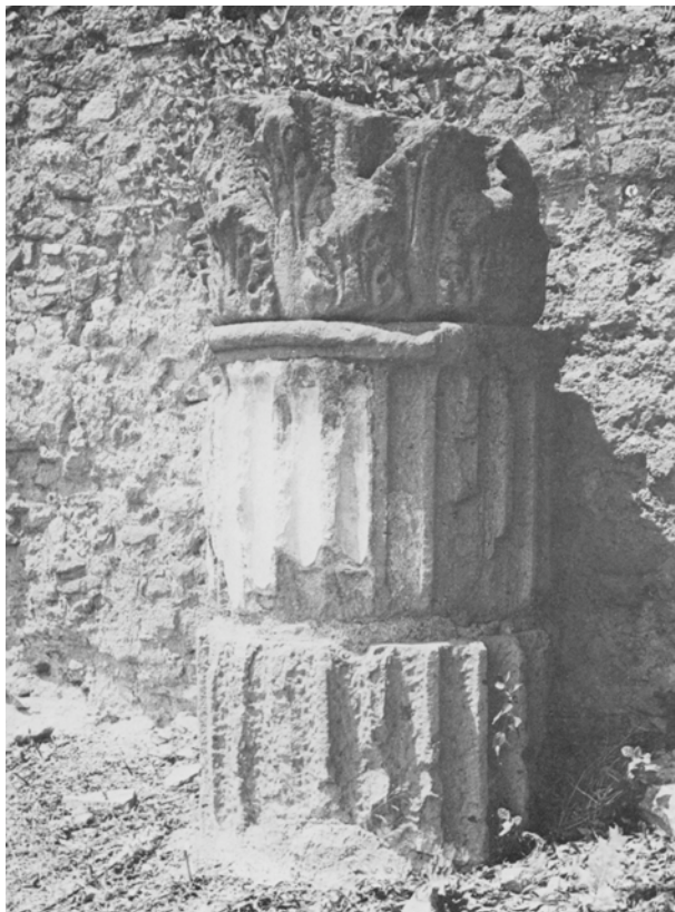
Figure 10. Column with stucco coating from the Augustan metroön. Southwest Palatine, Rome. Photo: CCCA III : pl. VII.
